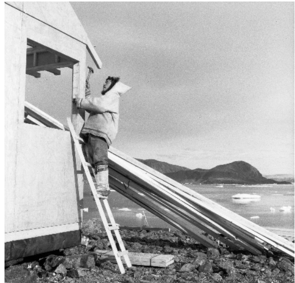
Inuk Special Constable Minkyoo of the Twin Glacier Detachment of the RCMP erects the building for the post at Alexandra Fjord, Nunavut, 1953. Source: Library and Archives Canada/National Film Board of Canada fonds/a137757.
